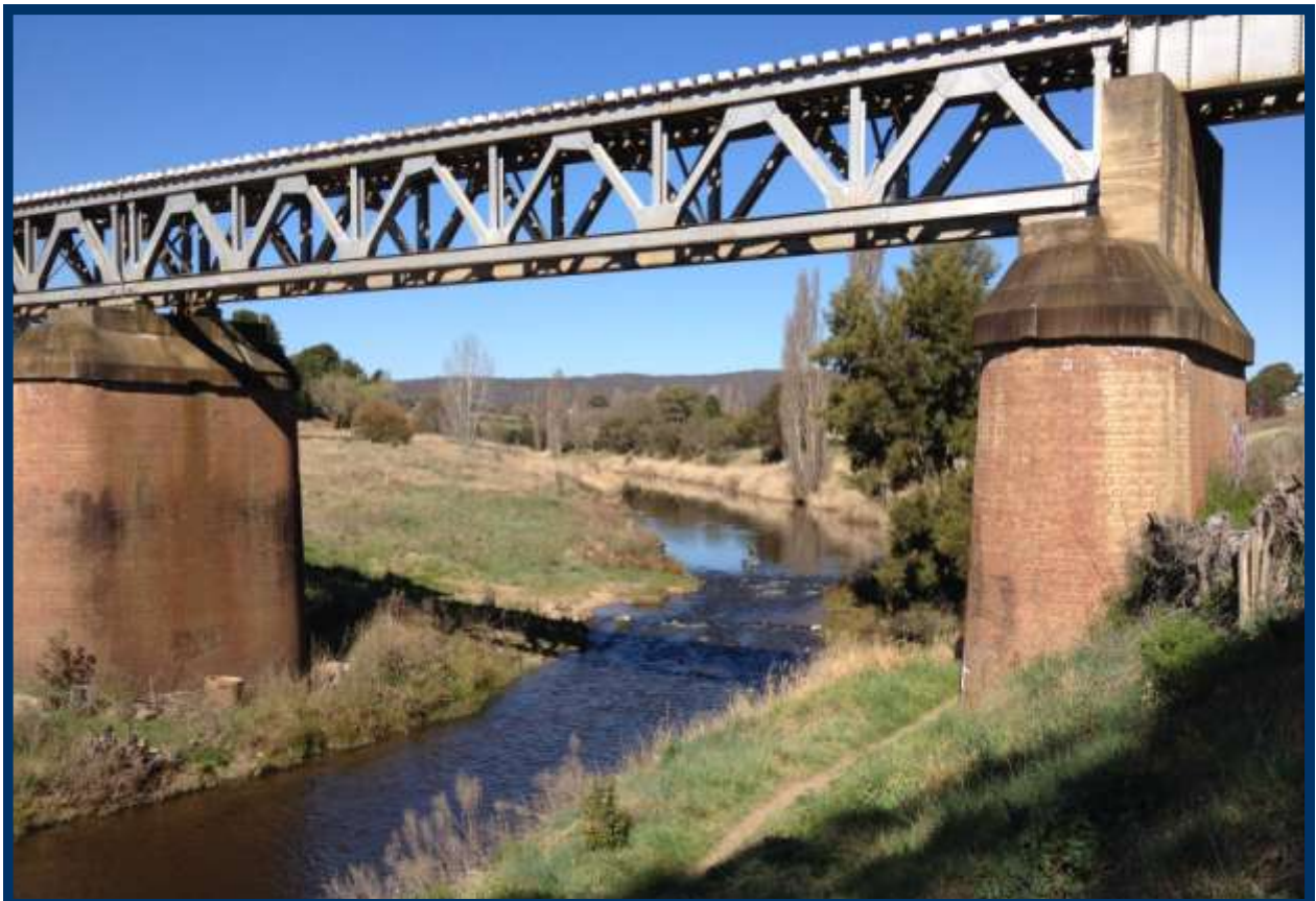
Railway crossing on Queanbeyan River.
